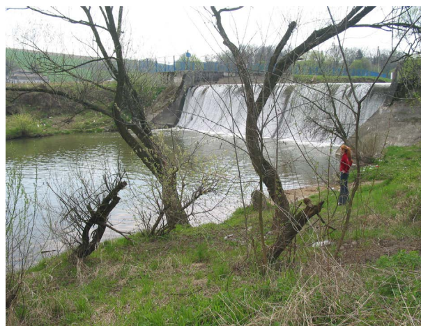
Figure 2. Uszwica River in Brzesko. The 5.3 m high weir built in 1913 was not equipped with any device for animal migration until 2020 [photo by M. Klich, 20.04.2004]
