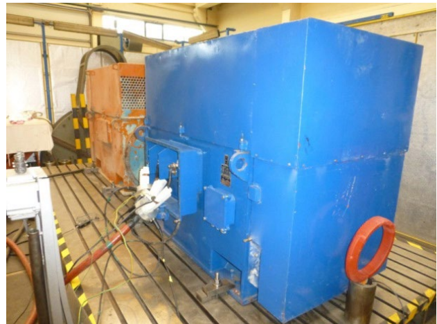
Figure 4. View of the stand for measuring high power HV machines with axial flux measurement
